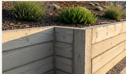
SLOPE · RETAINING WALL
